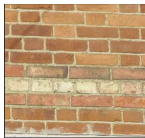
Buff coloured brick string course
