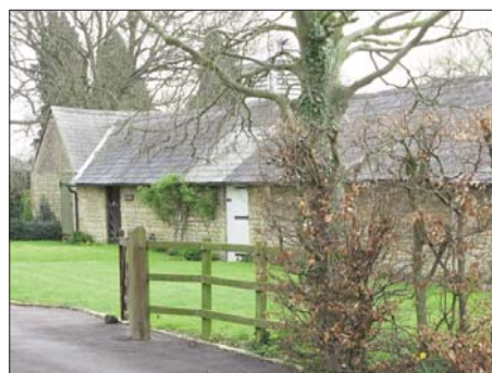
19th century ranges at the Old Manor House
