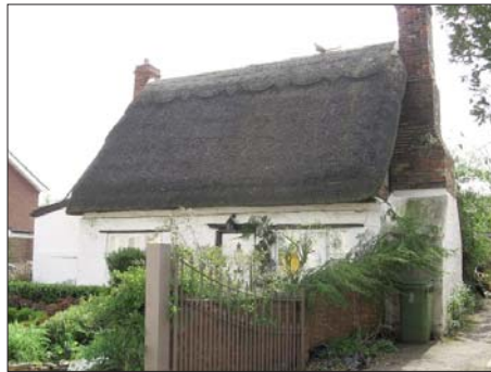
Old House Cottage, Main Street
