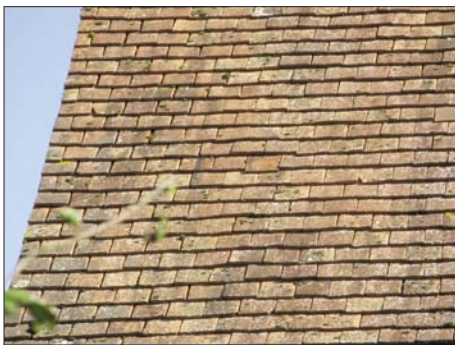
Traditional tiled roof
