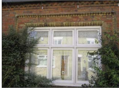
Brick hood mould
