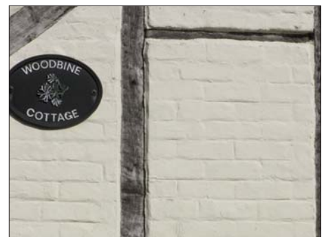
Painted brick infill panels
