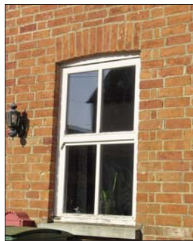
Brick segmental arch
